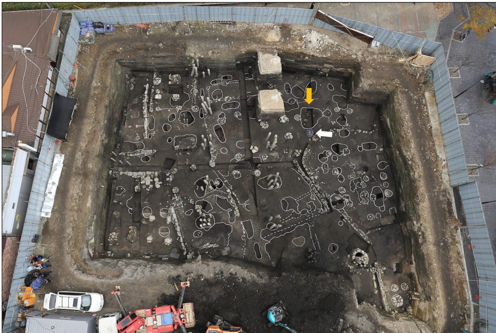
Figure 2 The excavation site at Gongpyeongdong site. Cattle and horse bones were collected at the 15 th century pits #1 (white arrow) and #5 (yellow arrow) situated at the layer VI of the excavation site.
